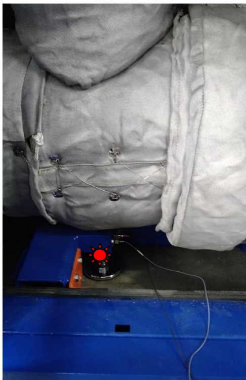
Fig. 9.16. D3 Measurement point D level 3 measurement base of the unit frame
