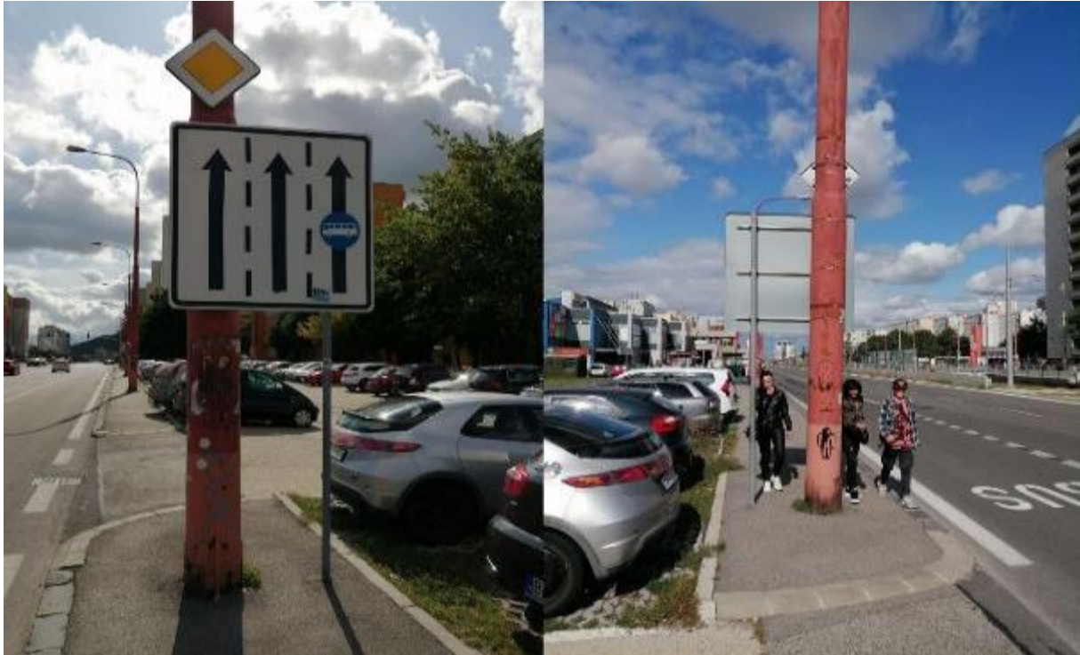
A picture 12-2 Improperly placed public lighting pole and traffic sign carrier (Source: Processor)
