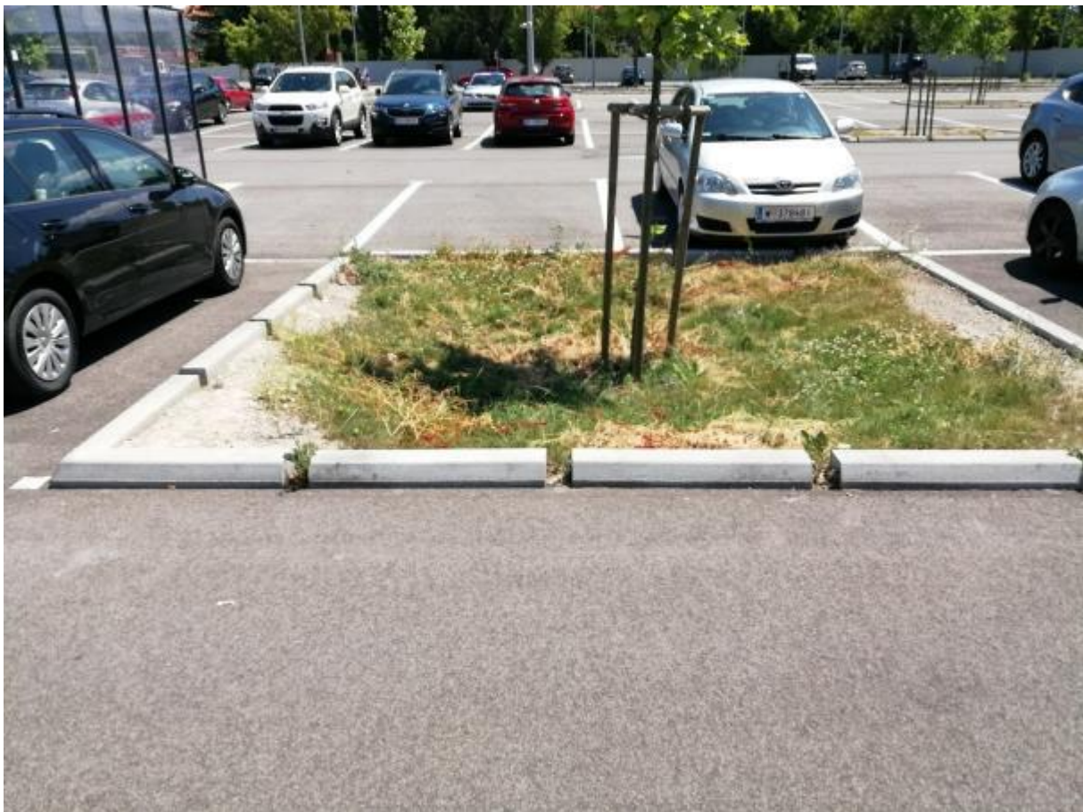
A picture 15-13 Drainage of the car park into the infiltration pit with greenery (Source: Processor)
