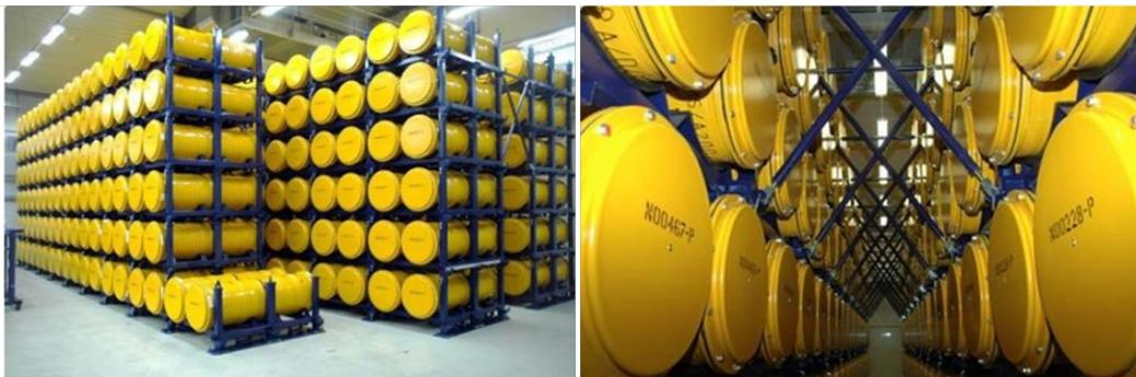
*Figure 5: Interim storage of the conditioned 200 litre drums*
