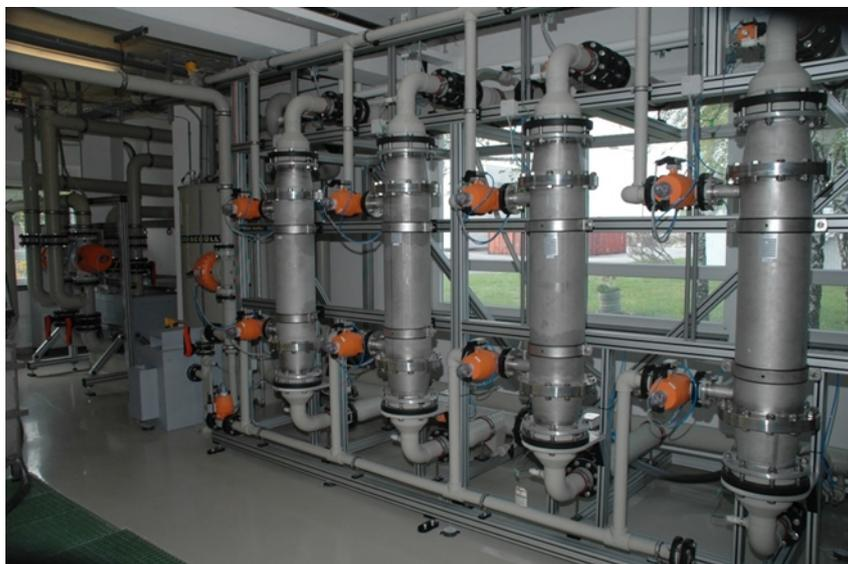
*Figure 6: Filtration unit of the ultrafiltration system*
